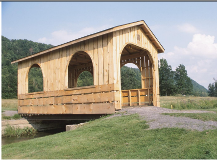
Bridge Timbers and Materials
