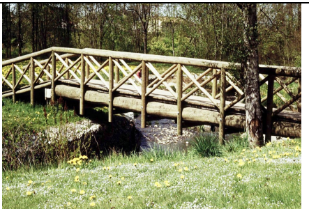
Foot Bridge Posts, Supports, Beams, Handrails, and Decking
