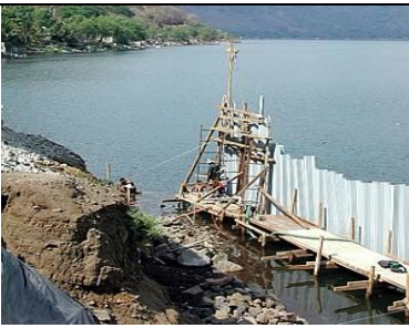
Commercial Bulkhead in El Salvador
