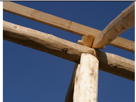
Framing Poles & Timbers
