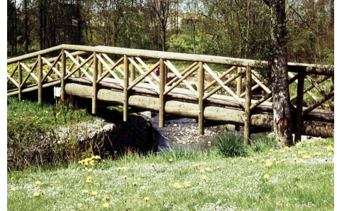
Treated Bridge Timbers & Poles
