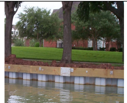
Vinyl Sheet Piles & Treated Timber Front Wale
