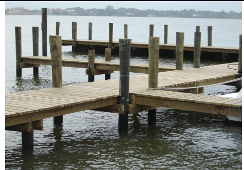
Treated Pilings & Decking
